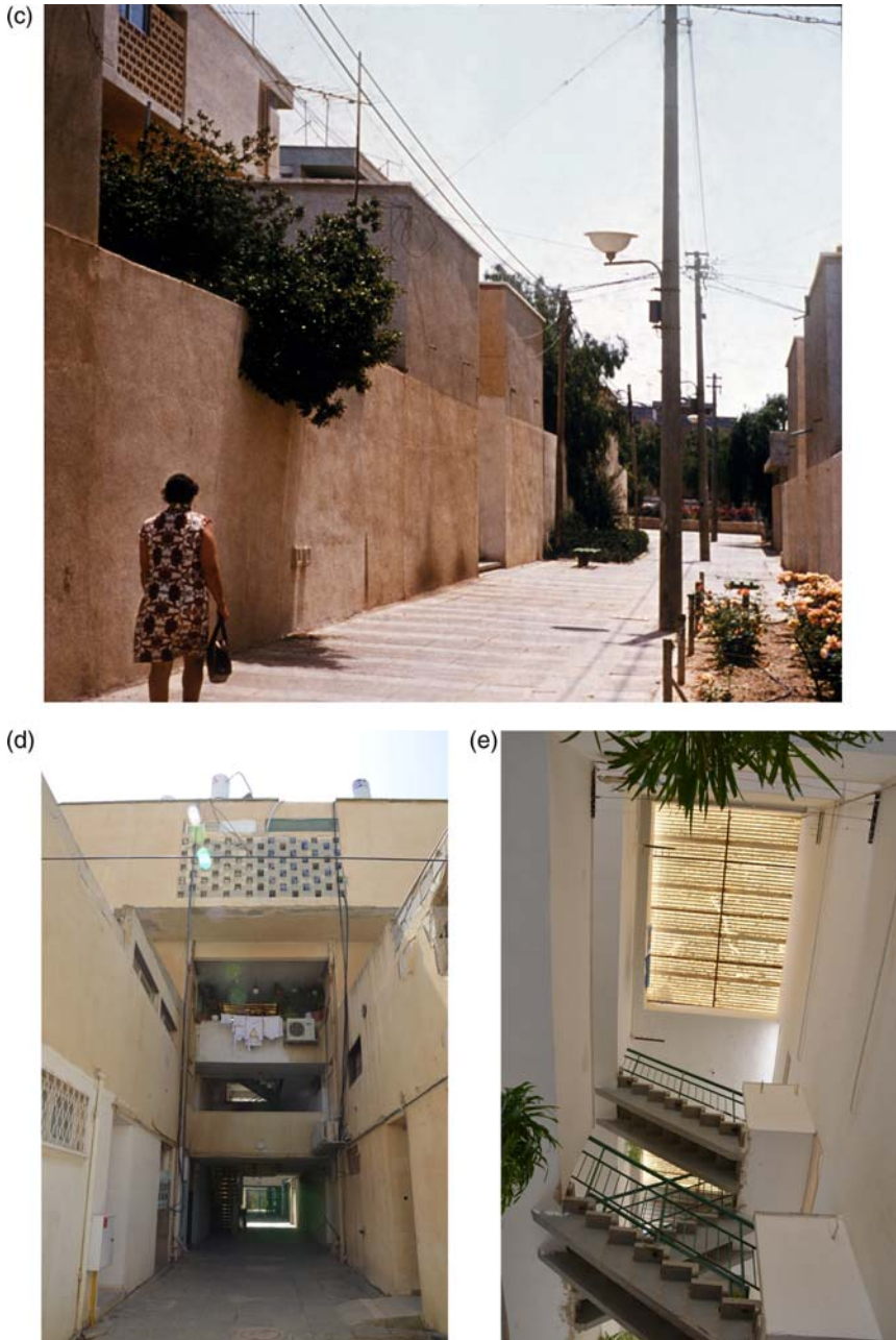
Figure 7. The Patio Houses in Arad. (a) A distant view of the Patio Houses in the early years. From Israel Builds 1967: New Trends in Planning of Housing (Jerusalem: Ministry of Housing, 1967). (b) An illustration of the Patio Houses cluster. Digital drawing by Asaf Yossefian and Hadas Nezer. (c) The view from the alley along the rows of adjacent Patio Houses. Photo by architect Ilana Elrod. (d) The view from the “patio alleyway.” Photo by author. (e) Looking upwards at the full height of the patio space through the stairwell. Photo by author.
